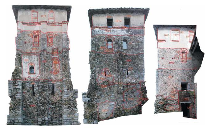
Picture 6: The analysis of the elevations and surveys aimed at the realization of the photo rectification of the structures (Archaeological Park of Castelseprio and Torba)
