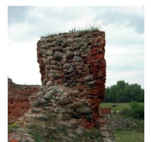
Photo9. Degradation of the wall due to the environmental factors /Międzygórz castle/
