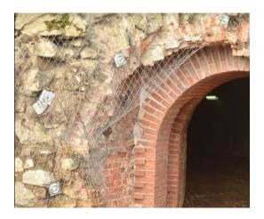
Photo17.Protection of the damaged wall's face with a steel mesh mounted by the anchors (photographer - Grzegorz Basiński)
