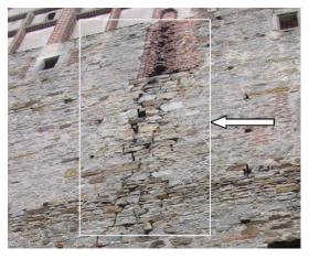
Photo13.Damage to the masonry structure /castlein Drzewica/
