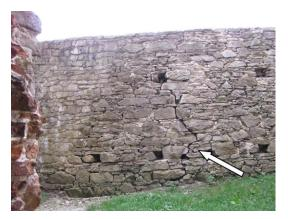
Photo12. Damage caused by uneven settlement /Krzyżtopór castlein Ujazd/
