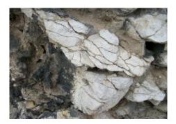
Photo10. Cracking of a masonry material /castle in Rabsztyn/
