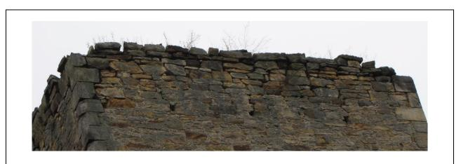
Fig. 12.Degradation of the crest of a stone wall constructed of a really durable material caused by the effect of rainfall and snowfall.
