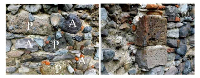
Fig. 2 Building material of the cloister (Cistercian Abbey): A - andesite, P - pyroclastic material
