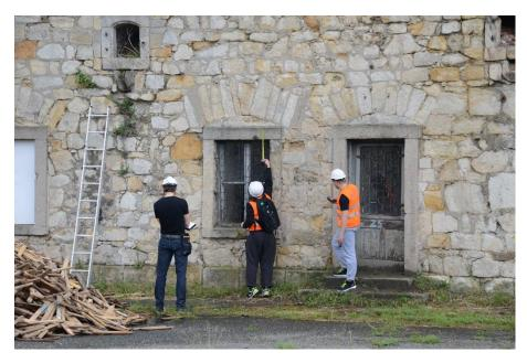
Photo 1 Measurements of the Donjon facade on the Kłodzko Fortress using the traditional method.
