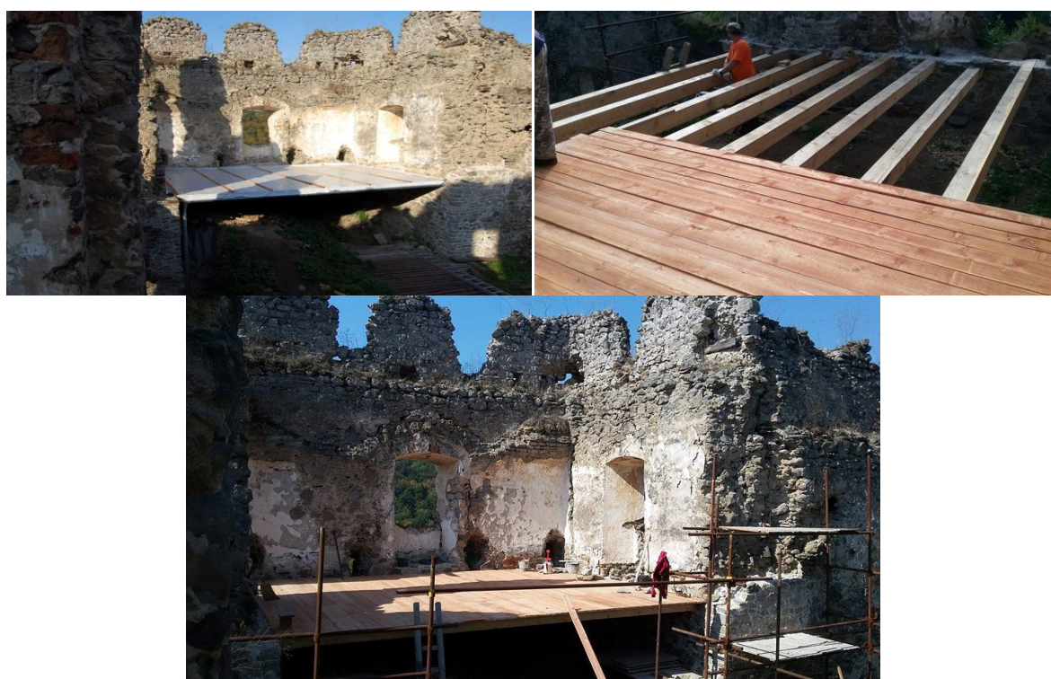
Figure 57 Roof on the defense tower of Castle Čabrad imitating a perished beam ceiling protecting original construction of the vault of the ground floor and redirecting the precipitation waters from the foot of the walls (it was causing a slow sliding of the tower)
