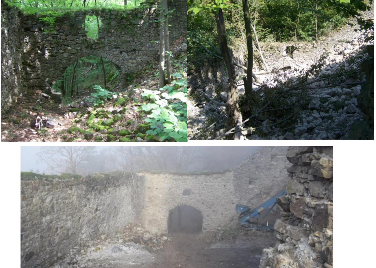
Figure 60 After a large portion of the ramparts of the inner part of the castle collapsed and filled the outer courtyard with rubble, it made the entrance gate impassable. Since there was no other access, the cleanup of the rubble had to be performed by hand, whi
