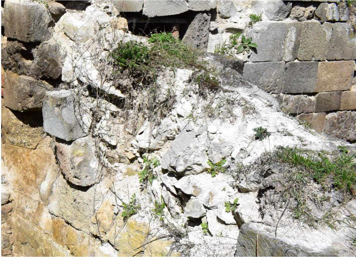
Figure 30 Detail of modern mortar
