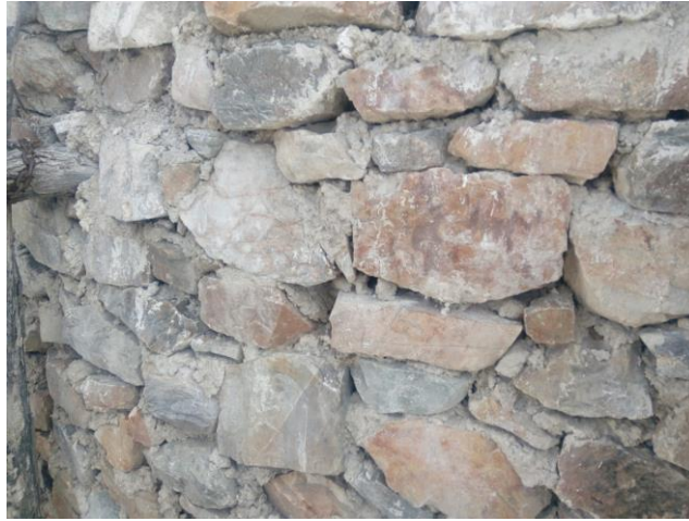
Figure 63 As the workers employed by the project are rarely professionals, they have no experience in the work they are hired for. This can undermine the professional work, and result in poorly executed craftsmanship. An example is this piece of masonry with no e
