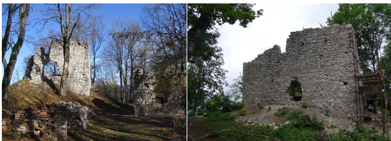
Figure 59 Restoration of the main tower of Castle Muráň which was done without any interference with the buried parts of walls. No details were recreated. The openings in the walls with unknown original shape were left in the form of cavern, only the masonry arou
