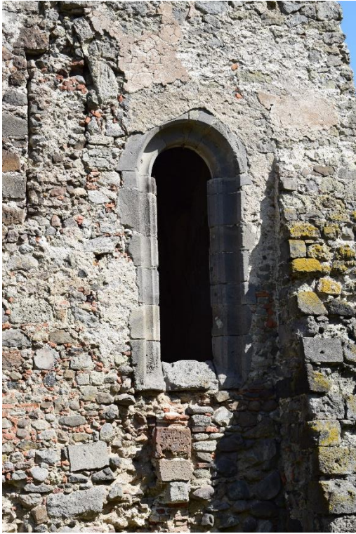
Figure 23 Gothic window with a tracery from the extinct church, secondarily reassembled during the conversion of the sacristy into a chapel
